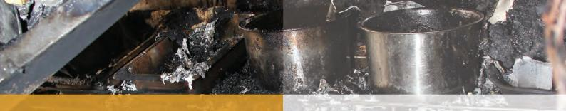
In April 2016, a coffee shop in Jurong West was engulfed in flames. The small fire started in a stall and quickly spread to several other stalls through the oil accumulated kitchen exhaust duct. As a consequence of the fire, the coffee shop was closed for weeks resulting in business disruption to all its stall owners.
